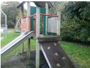
The unit is easily accessible and has an opening in the barrier to steep play elements in excess of 500mm Finding:
