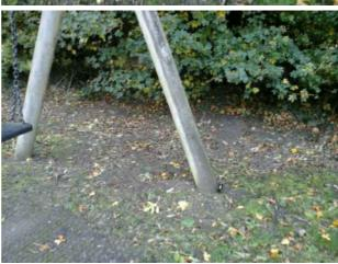
The timber on this item has severe rot in a support post Finding:
