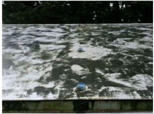
**Finding:** There is/are bolt cap covers missing or damaged bolt cap covers damaged on the item
