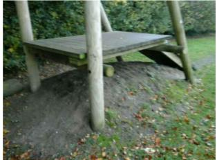
Finding: The surface has eroded in some areas Action: Reinstate the surface
