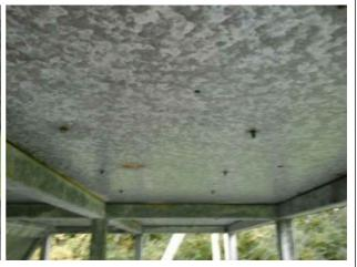
Finding: There are sharp protrusions beneath the item **Action:** Remove the sharp protrusions
