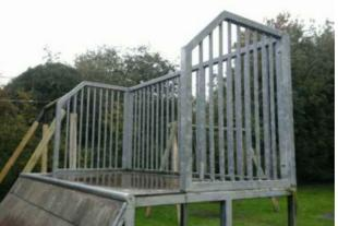
The height of the barrier is less than 1200mm  $\,$  Action: and fails the requirements of BS EN 14974  $\,$ Finding:
