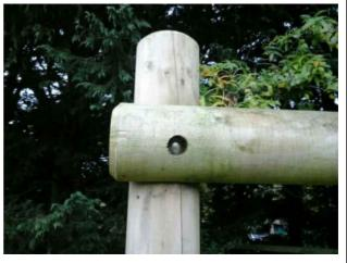
There is/are bolt cap covers missing or damaged on the item Finding:
