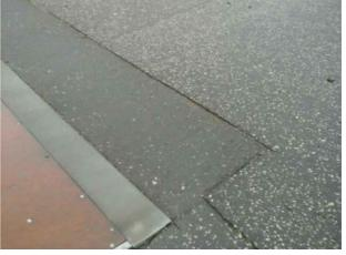
Finding: There is vertical height difference on the rolling surface in front of the kicker plate of
