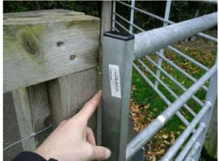
**Finding:** The opening between the gate and the post is **Action**: less than 12mm and could trap users fingers
