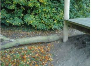
A tree is within the falling space of the starting platform Finding:
