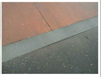
Adjust height to ensure a maximum of 5mm change in level Action:
