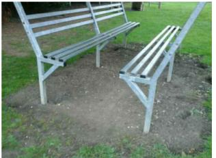
The area around the shelter has eroded and may become slippery Finding: Action: Reinstate eroded area
