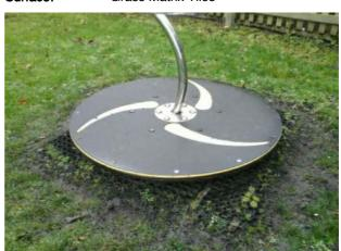
The bearing on the unit is dry and item difficult to rotate Finding:
