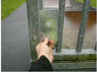
The horizontal opening in the barrier is in excess of 89mm and fails the requirements of BS EN 14974 Finding:
