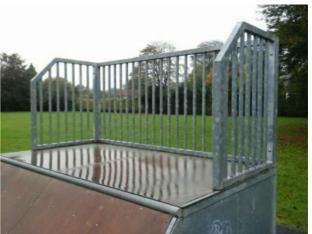
The height of the barrier is less than 1200mm Action: and fails the requirements of BS EN 14974 Finding:
