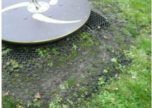
The grass mats are silted up and the soil is compacted; this may have an effect on the impact absorbing properties of the surface Finding:
