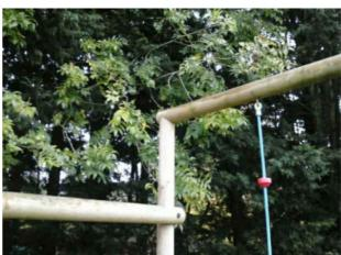
Finding: The tree canopy overhangs the equipment and is less than 2.0m away
