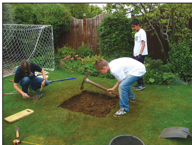
Using a mattock safely and effectively.
